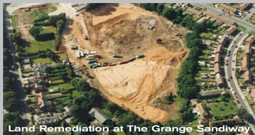
Land Remediation at The Grange Sandiway
